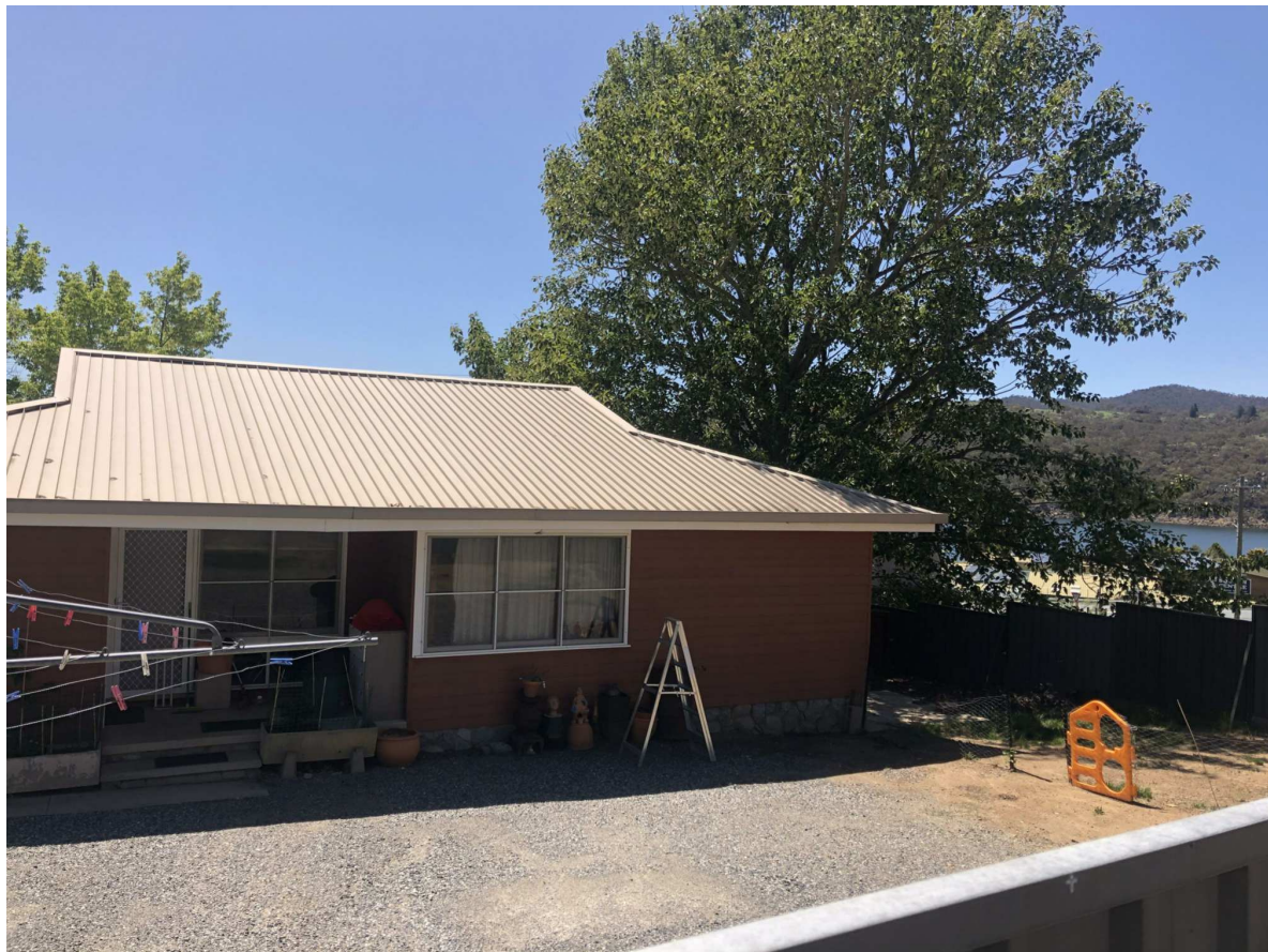
6. EXISTING POLICE RESIDENCE
