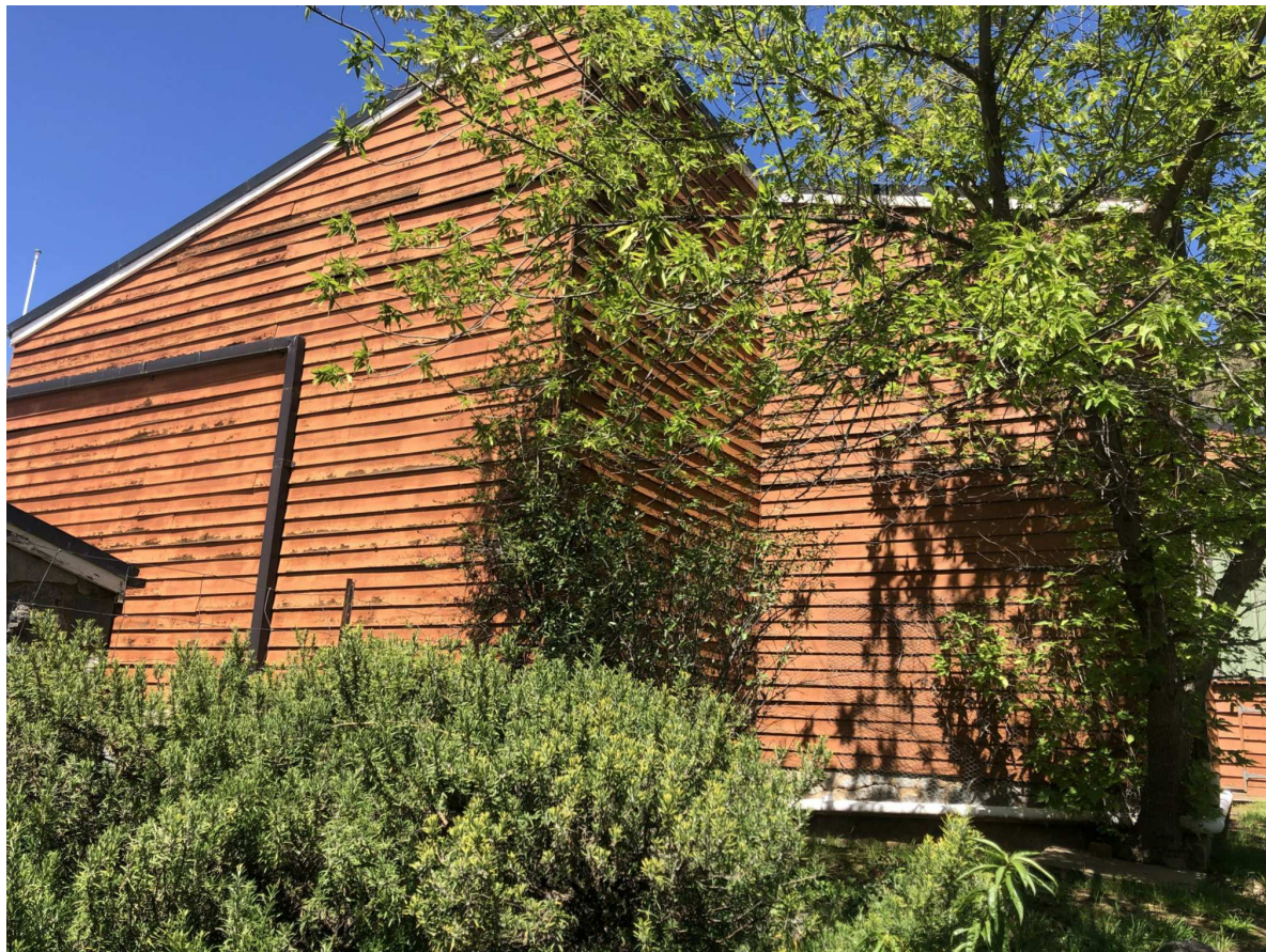
9. EXISTING POLICE RESIDENCE
