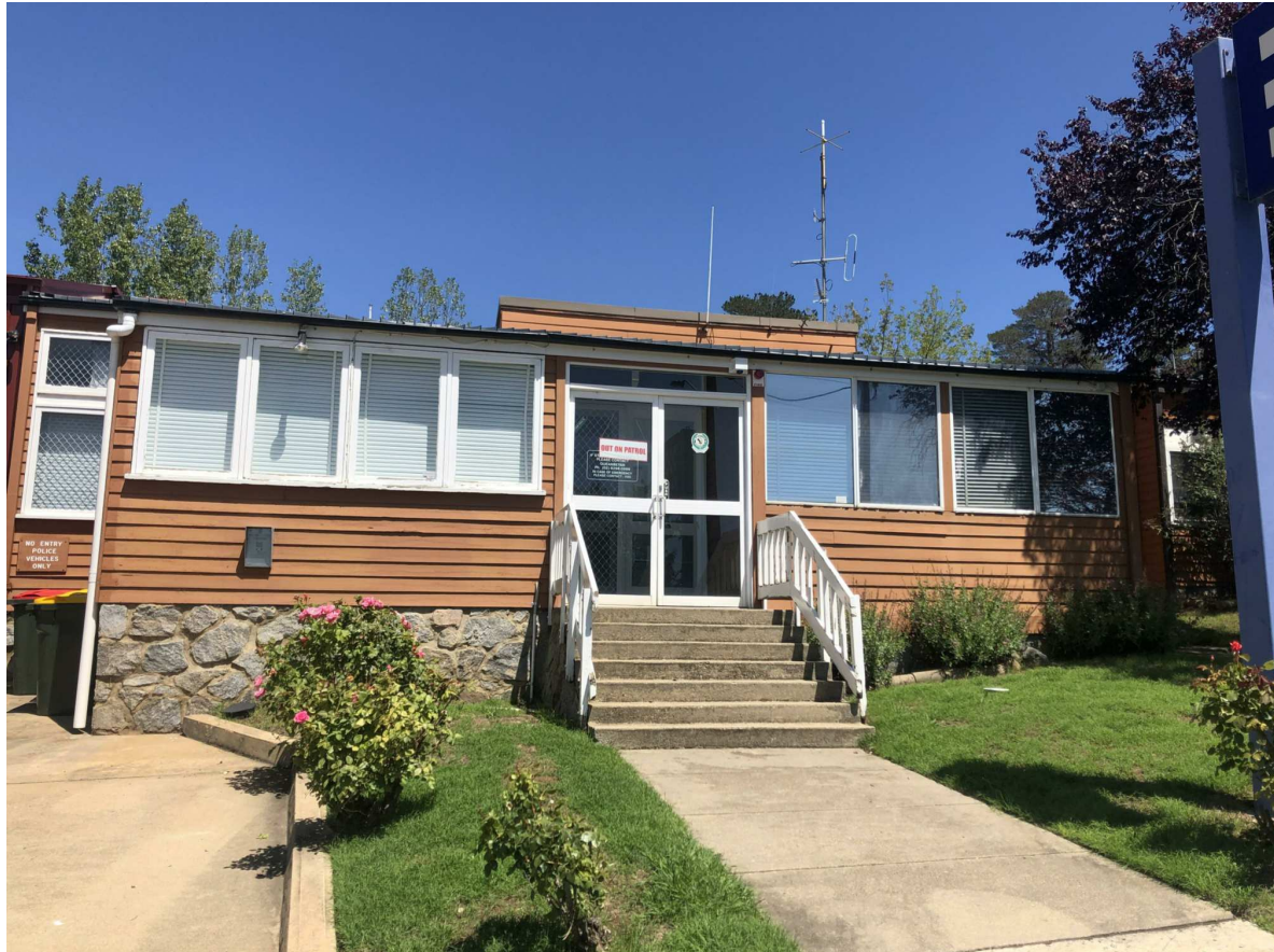
2. STREET FRONTAGE OF EXISTING POLICE STATION ON THREDBO TERRACE
