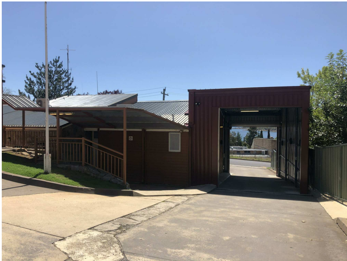
8. EXISTING VAN DOCK VIEWED FROM SOUTH
