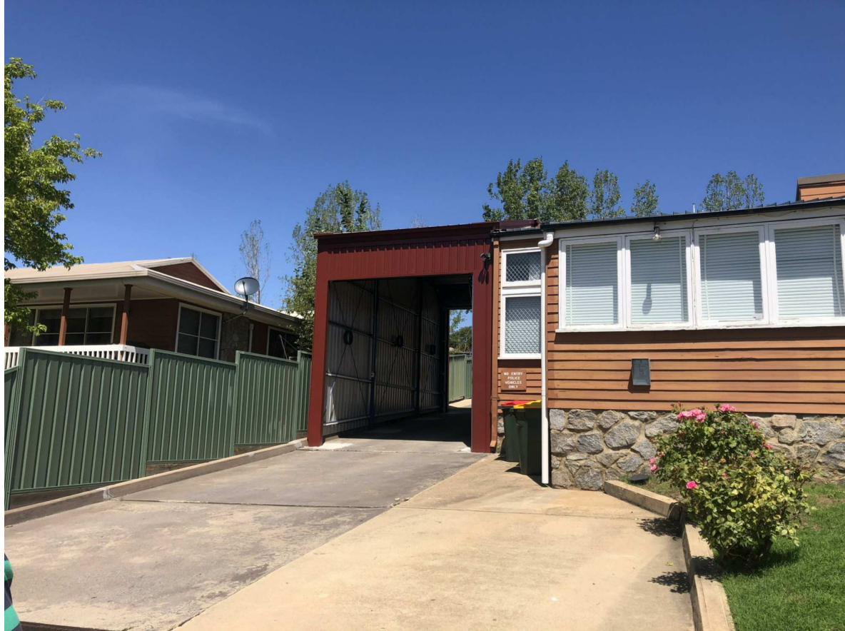
3. EXISTING VAN DOCK & VEHICULAR ACCESS FROM THREDBO TERRACE
